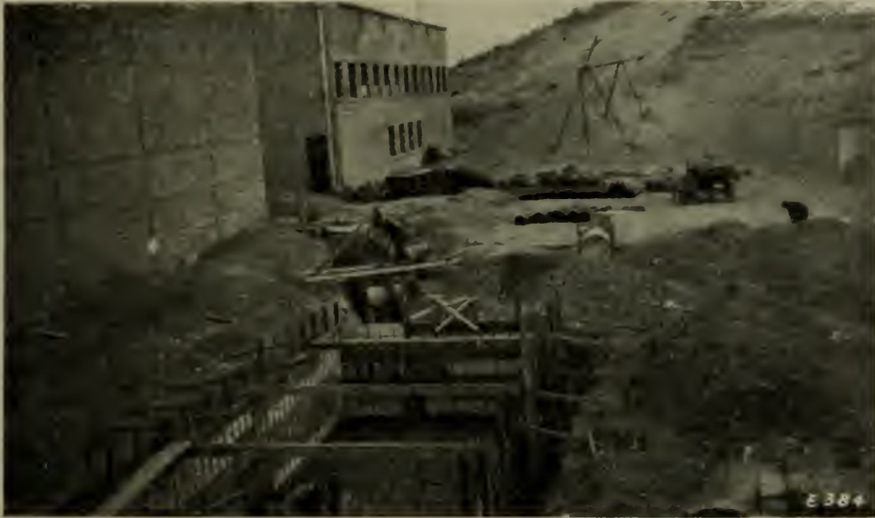
VIEW SHOWING CONCRETE SEWER PIPE.
